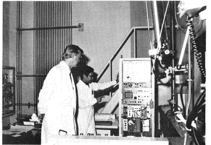
Suyama demonstrates automated control of the leached hull monitoring system.
