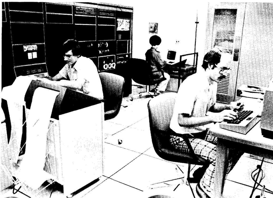
The NBL computer system processes data from NDA systems, performs numerical calculations, performs statistical analysis of laboratory measurement data and monitors the laboratory measurement quality assurance programs for uranium and plutonium assay
